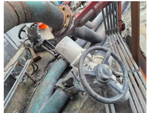
8" knife gate valves replaced in line.
